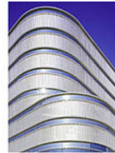
Veranda Parking Garage in Rotterdam, the Netherlands, designed by Architectenbureau Paul de Ruiter b.v. Photo: Rien van Rijthoven
