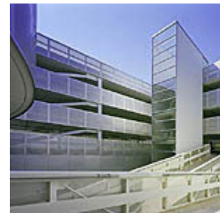
Interior courtyard extends down four stories below grade. Photo: Rien van Rijnhoven
